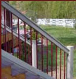
Powder coated heavy wall aluminum balusters are available in round or square profiles.
